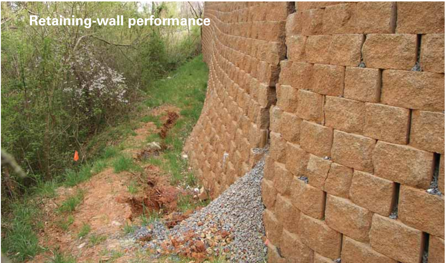
Photo 5 | Soft foundation soils left in place.
