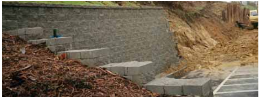
Photo 2 | Structural excavation protection during work.
