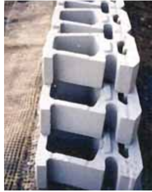
Photo 7 | Multi-stacking of SRW units.
